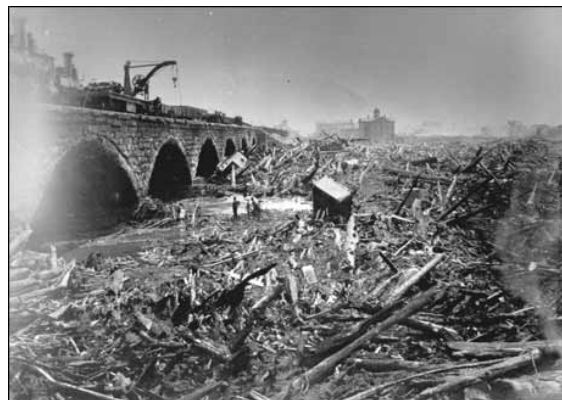
Debris at the train bridge
